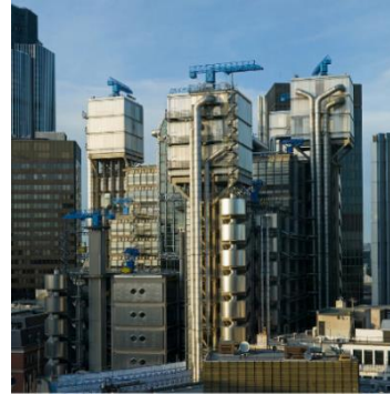
Lloyds Building, London
